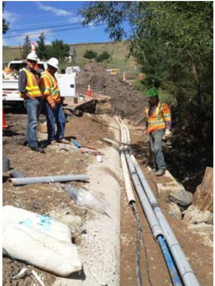
*CenturyLink technicians inspect lines damaged during 2013 Colorado flooding.*
