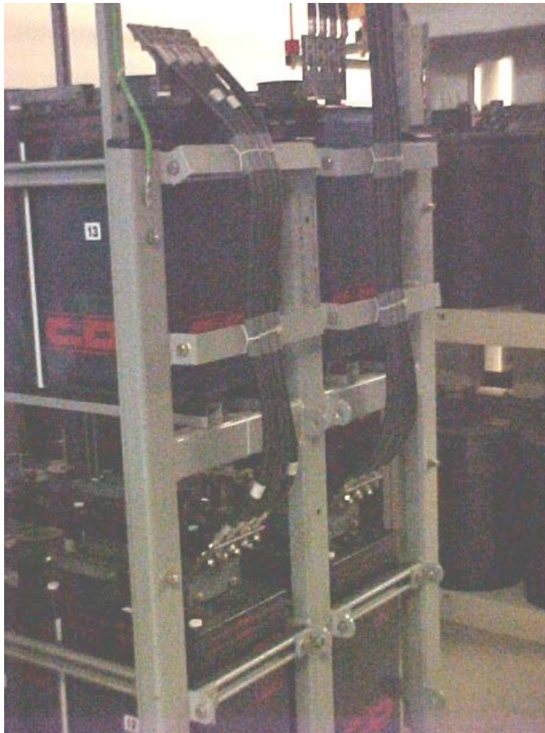
Figure 3-1: Typical Arrangement of Cables for a Flooded Battery Stand
