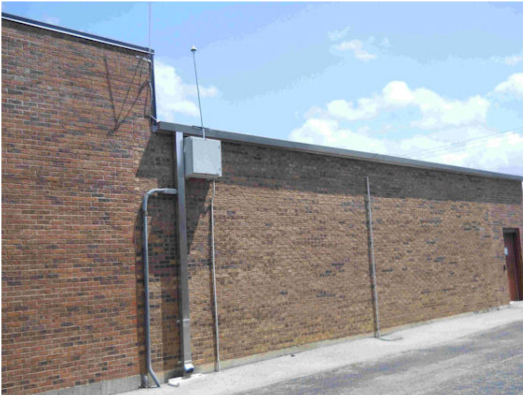
Figure 7-32: GPS Antenna Above Roofline Protected by Lightning Rod
