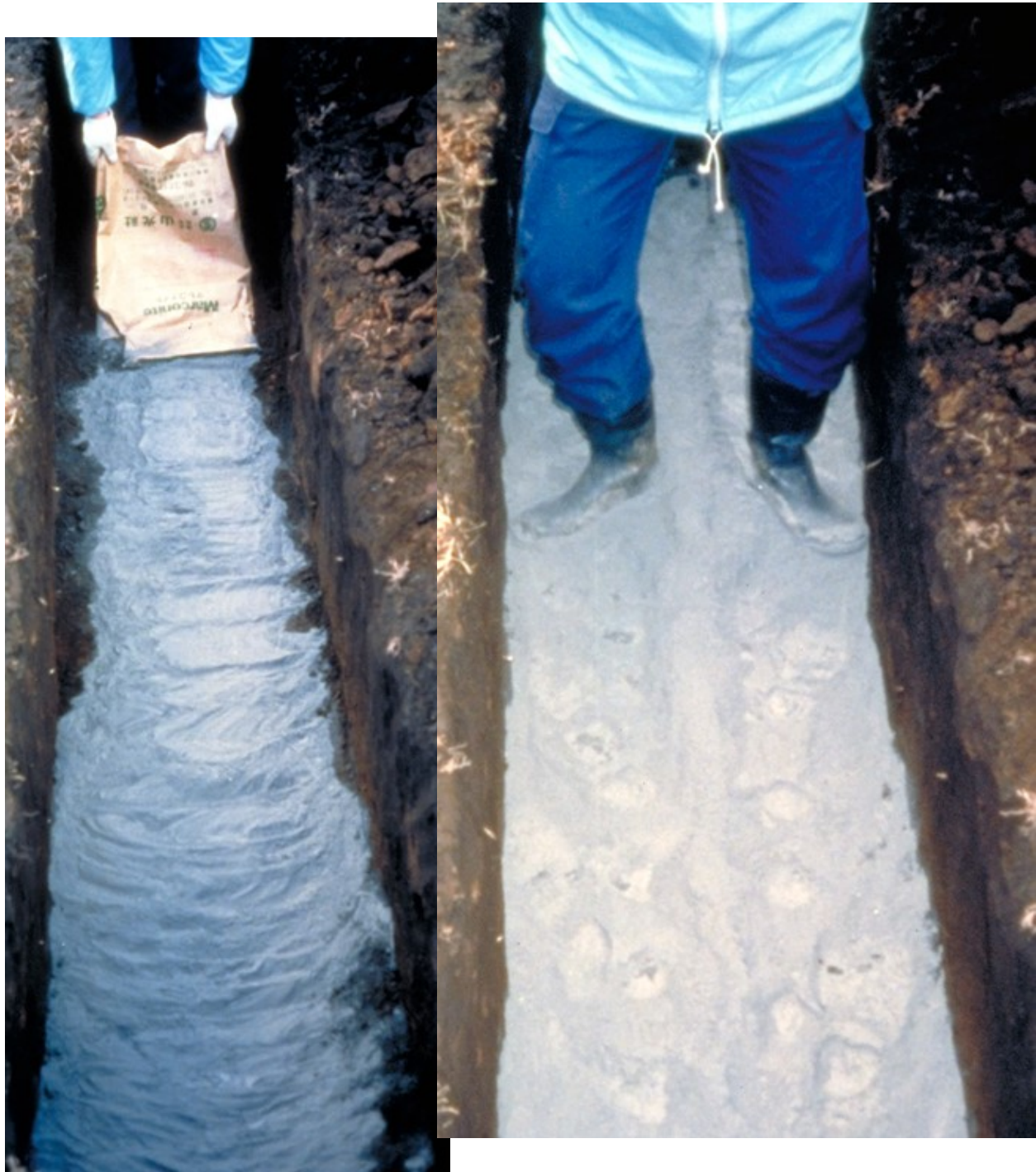
Figure 3-3 Lo-Ohm Concrete Installation
